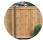
12 Perimeter board fence
